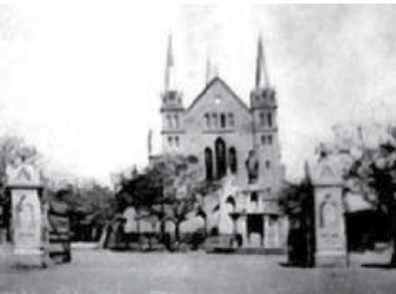
The St. Patrick's Cathedral - built in 1881. The first picture (dating from 1892) is a British Library image, also showing the St. Joseph's Convent School in the background (established in 1868)
