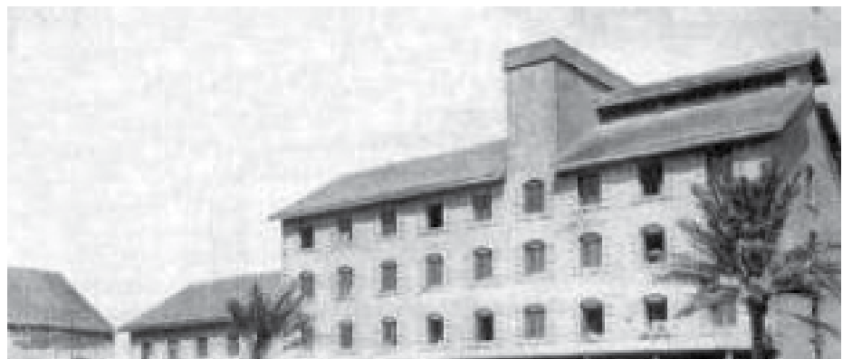
The Sindh Flour Mills and Warehouse (c. 1896)
